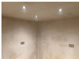
Finished walls & ceiling
